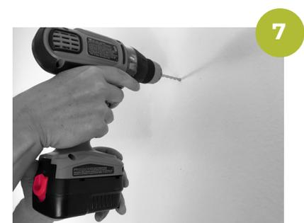
**7.** For the penciled dots that will take anchors because there are no studs, carefully drill a 1 ¼" deep hole into the center of each with a 5/16" drill bit. Careful! If the hole is too wide the anchor will not latch.
